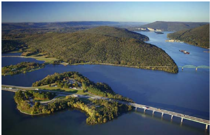
Interstate 24 crosses the Tennessee River, near Chattanooga
